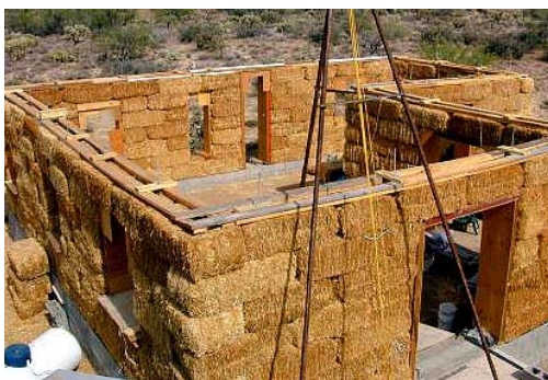
Figure 3: Load bearing straw bale house during construction
