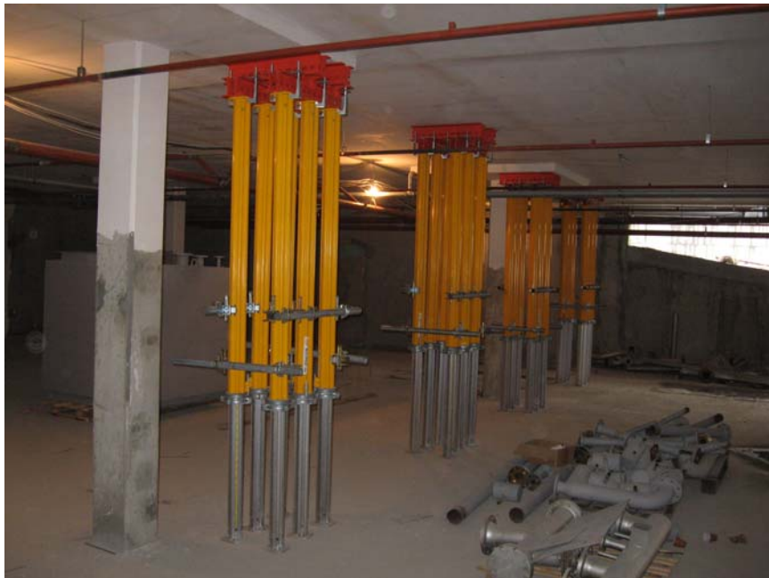
Figure 10. Shoring the supporting construction in the basement storey
