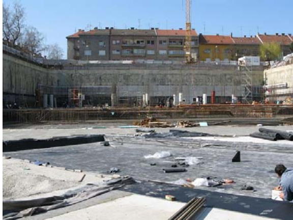
Figure 3 - View of foundation plate and sheet-pile wall
