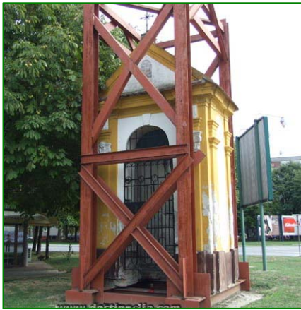
Figure 5 – Shifting the Chapel of Stone Cross
