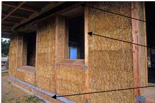
Figure 6: Wall of a light frame straw bale house
