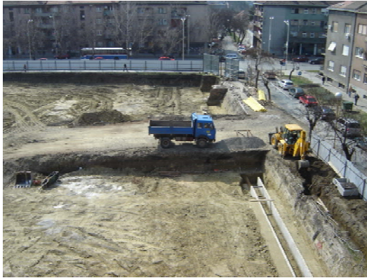
Figure 9 - Entrance and approach ramp to the excavation pit
