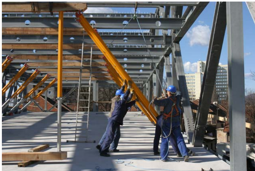
Figure 6. Shoring of superelevation of construction floors
