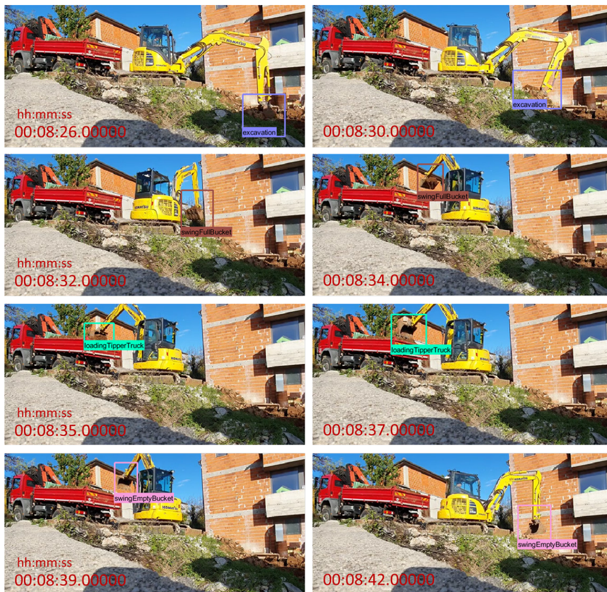
Figure 3. Examples of inserted labels for excavator working operation (image created by the first author)
