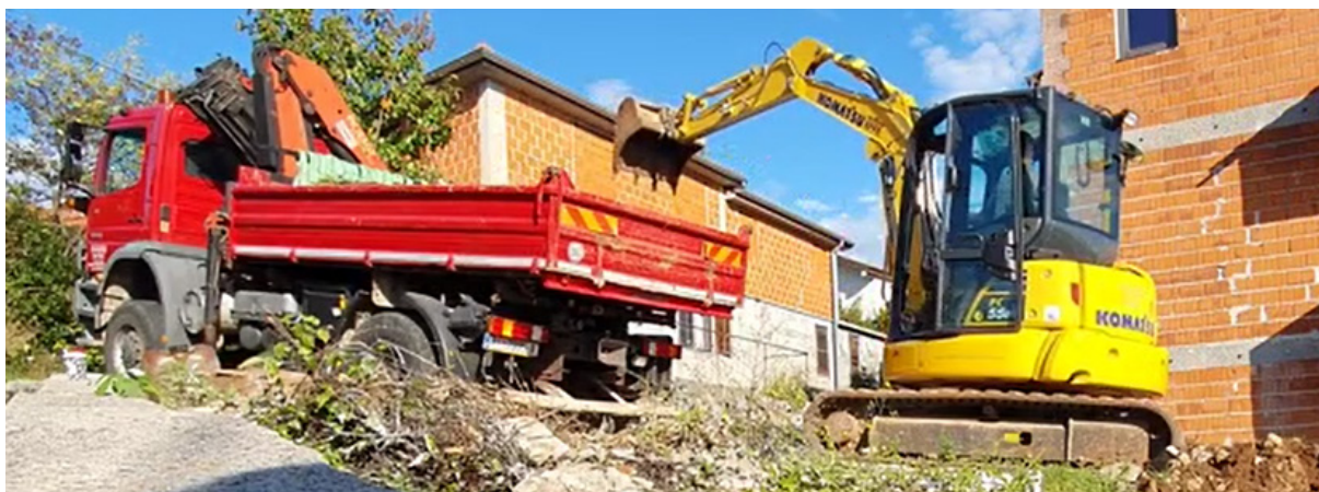
Figure 2. View of the used machines at the construction site in Matulji (Croatia) during earthworks (private album of the first author)
