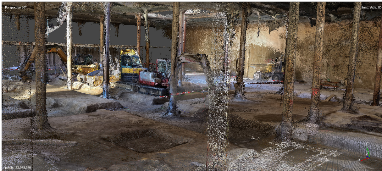
Figure 1. Dense point cloud recreating the excavation works under ground
