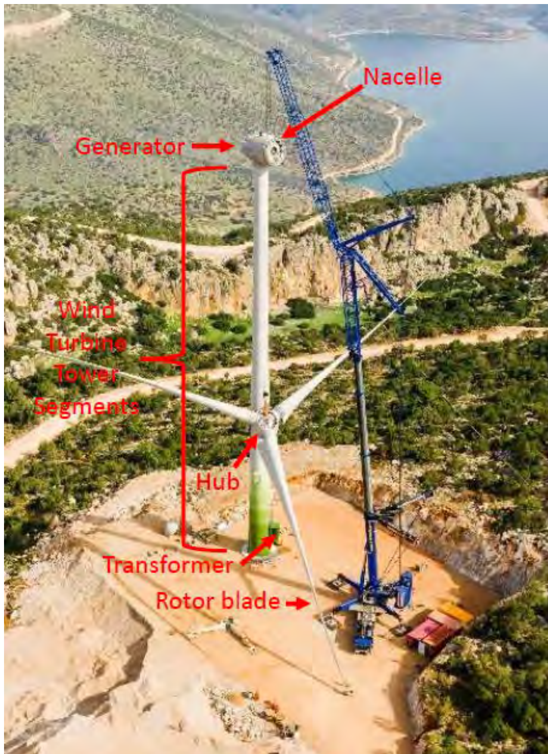
Figure 2: Wind turbine erection process
