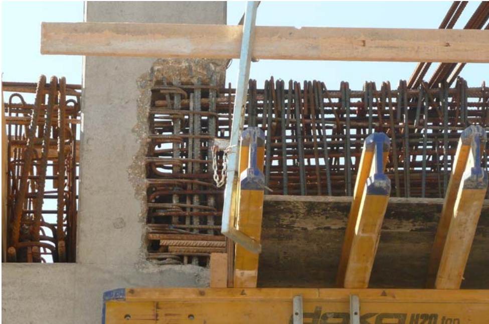
Figure 3: Due to poorly perfected project documentation mounting of monolith beam was impossible without additional processing of the precast element
