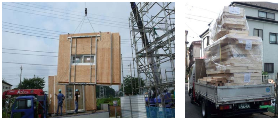
Figure 2: Pre-assembly at Factory (left) and Assembly at Construction Site (Right)
