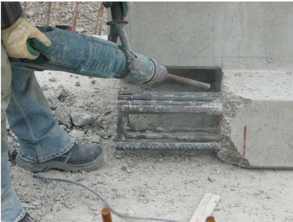
Figure 4: Poorly perfected project documentation resulted with a need to additionally process the precast element
