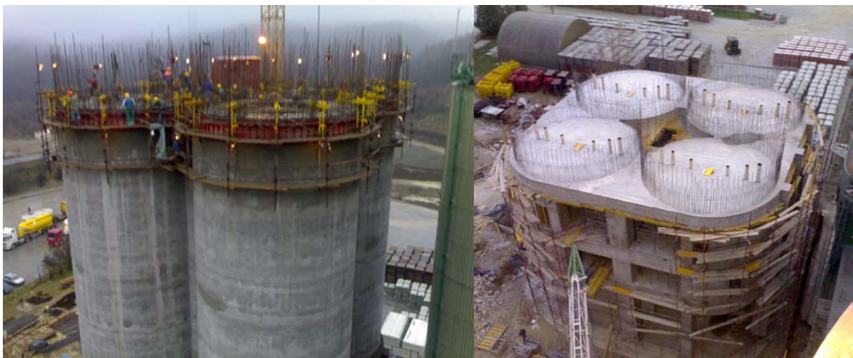
Figure 3: Chambers of the cement silo
