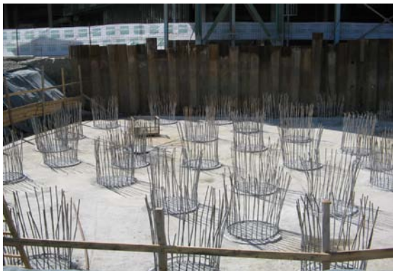
Figure 4: Reinforced concrete pilots
