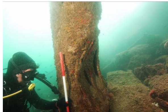
Figure 9: Damaged pier (cavitation impact)
