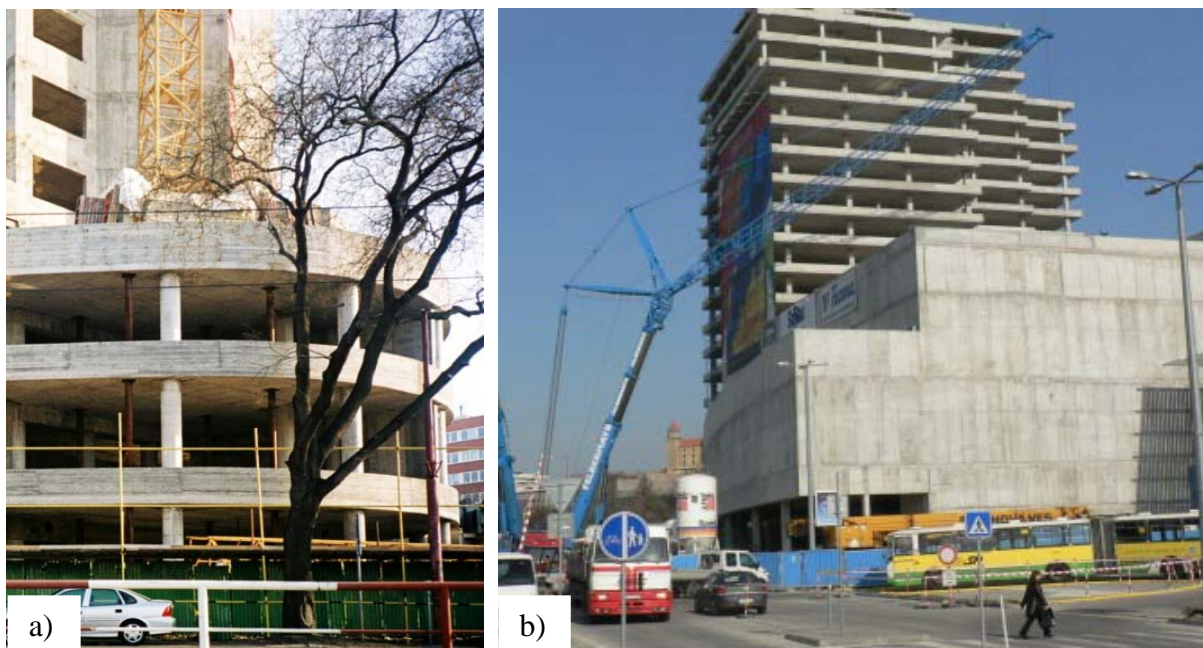
Figure 4: a) Crane on Ceiling Structure of the 3th floor – Gloria Bratislava, b) Removal of Crane Tower from Structure – Aupark Bratislava
